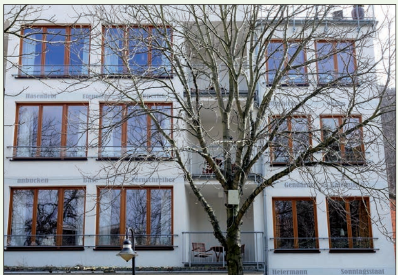
Kunst am Bau in Bad Harzburg.
